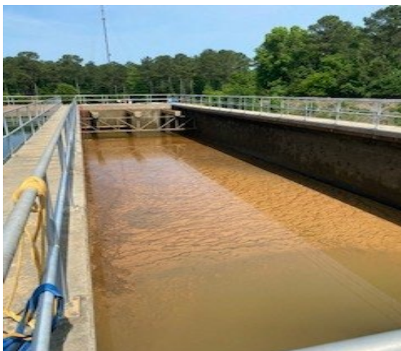
*Pictured left, almost 6 feet of sludge accumulated in less than 5 weeks due to the increased ambient air temperatures. Pictured right, cleaned sedimentation basin.
